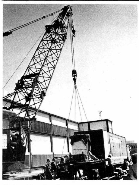
LIFTING the Cray's 10,500 pounds from moving van into the basement Computing Center at Sandia Livermore.
